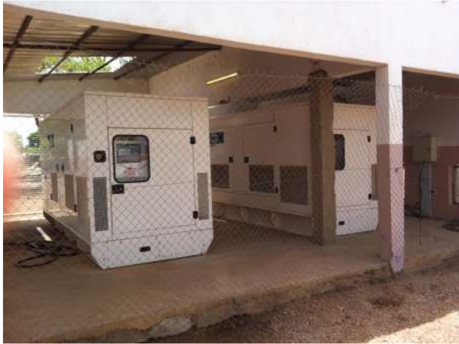
Figure 7: Douta Camp Diesel Genset Power Supply
