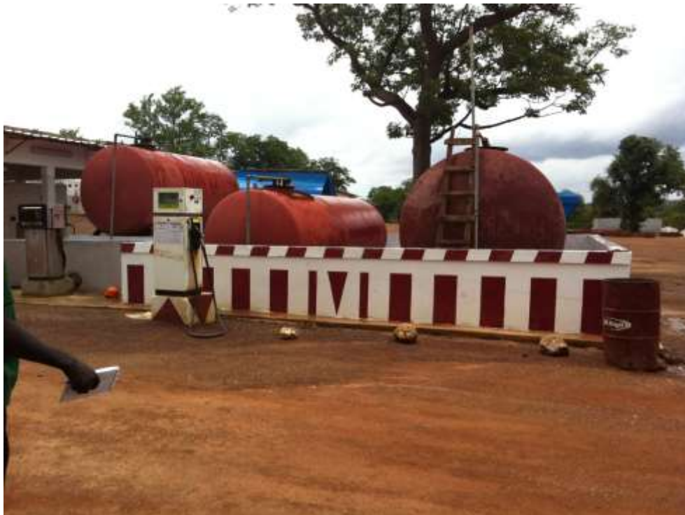
Figure 8: Douta Camp Diesel Fuel Facility – 85,000 Litre Capacity
