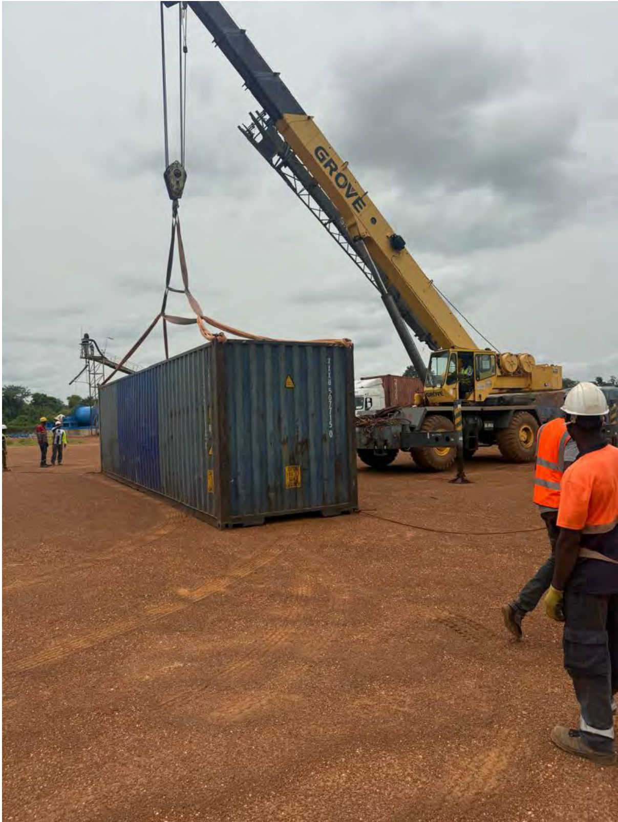
Figure 3 Motor Control Systems and Electrical switchboards shipped from Australia
