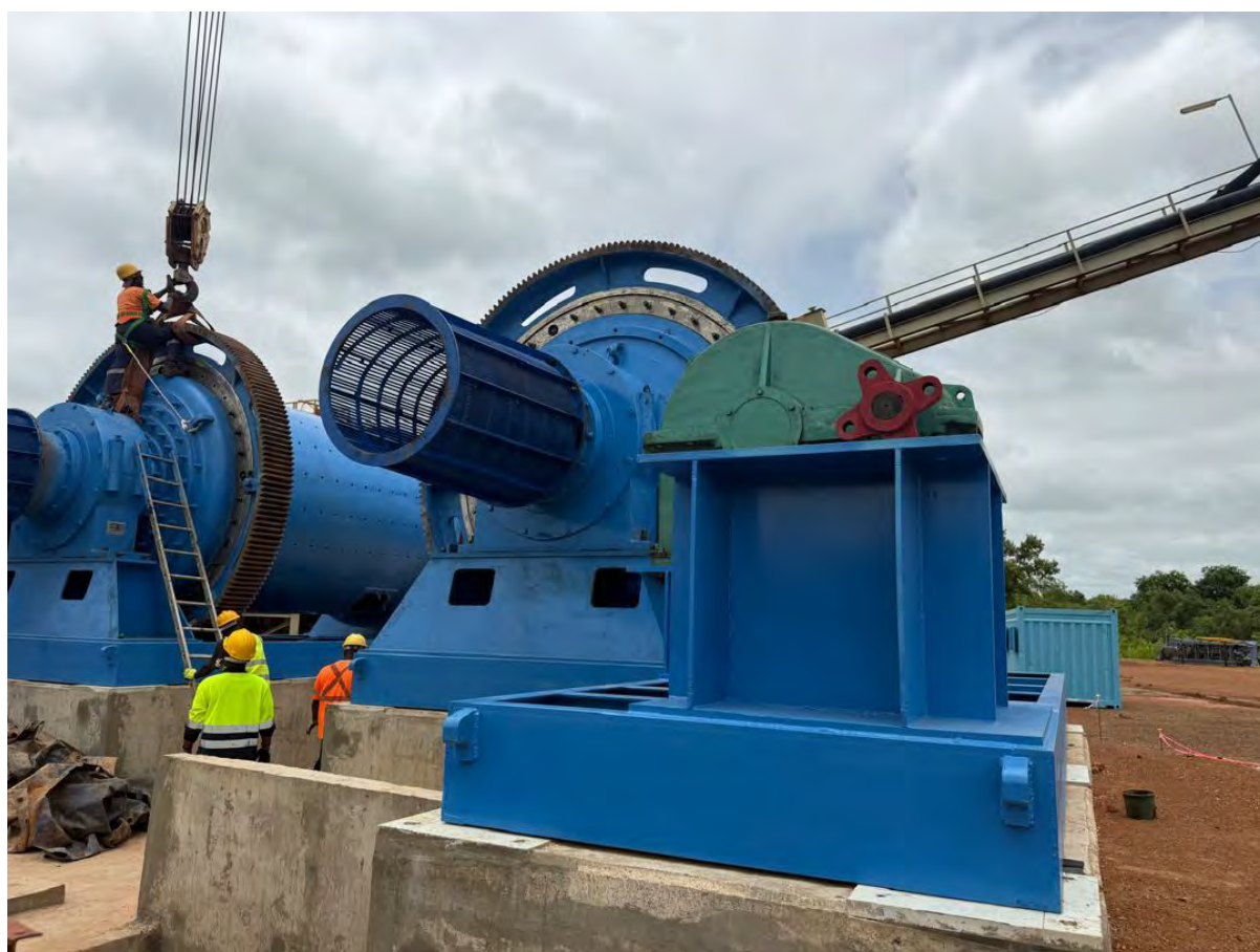
Figure 1. Ball mill installation at the Makabingui Gold Project
