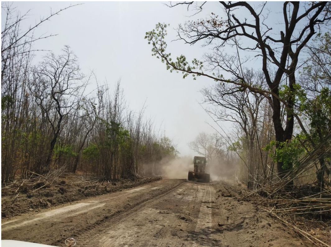
Clearing works for mine perimeter fencing
