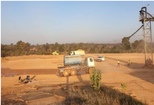
Site Preparation for CIL Plant Construction and Rom Pad
