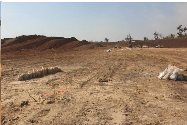
Ongoing Grade Control Drilling at Pit 1
