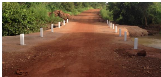
Road works completed
