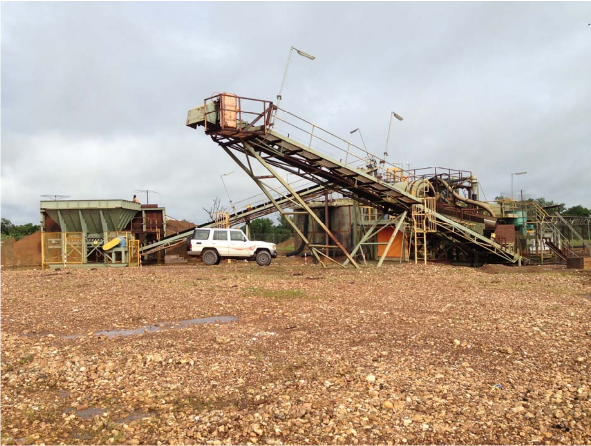
Figure 3 – Existing Gravity Plant
