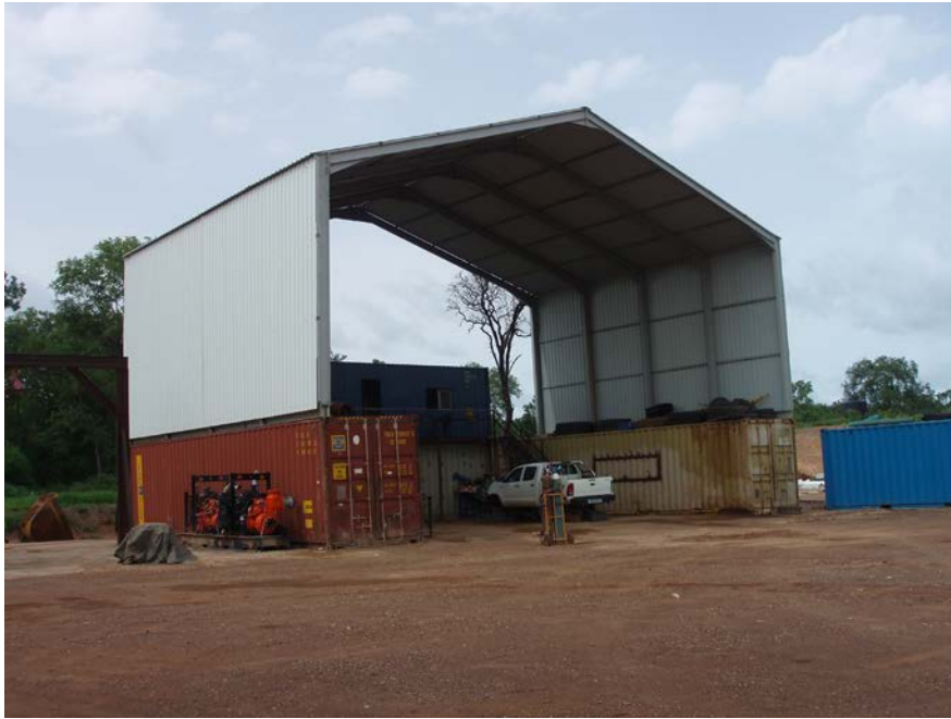
Figure 11 – Mobile maintenance workshop
