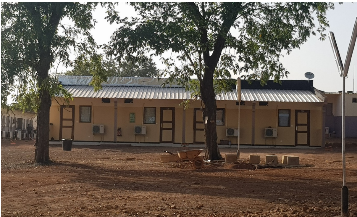
New accommodation block
