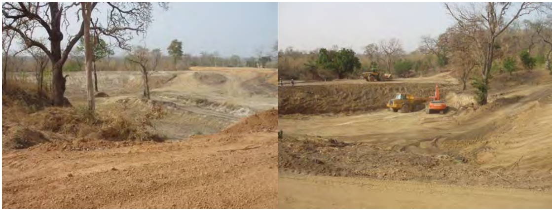
Figure 12 – Existing Tails Dam When First Constructed
