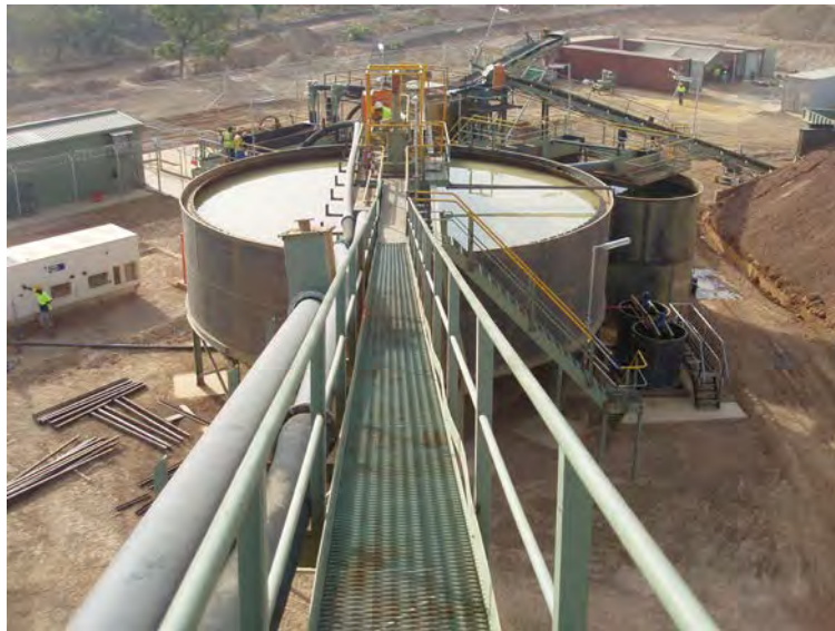
Figure 14 - View of gravity plant from 26 inch cyclone tower
