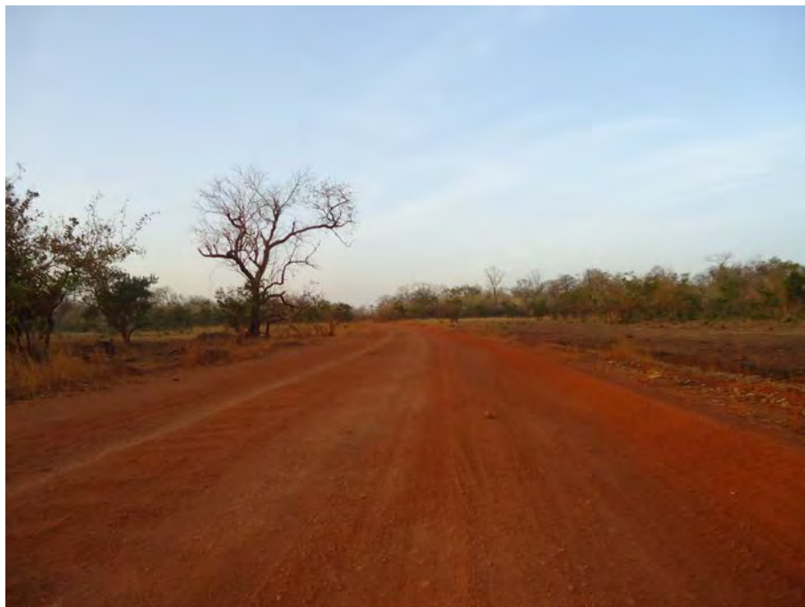
Figure 4 – Existing Road between Makabingui & Processing Facility
