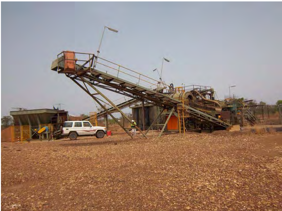
Figure 13 - Gravity Plant Located at Douta – 300ktpa Capacity
