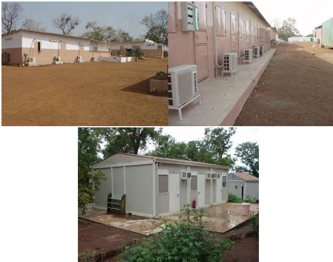
Figure 15 – shows sections of the 120 person Douta Camp, which includes offices, kitchen/dining hall, laundry and ablution/shower block. Within the camp compound there is a core shed, core cutting facility, light vehicle maintenance workshop, water sterilisation plant, fuel storage facility and medical centre.
