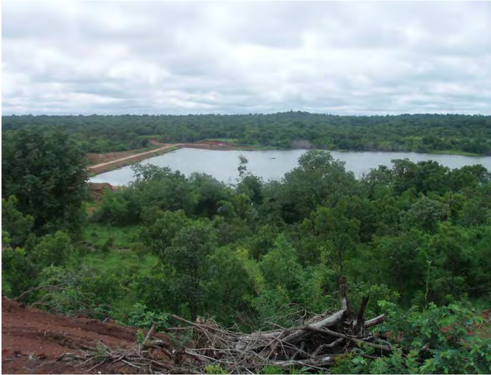
Figure 16 – shows the water storage dam (~500 Mega-litre) used for water supply to the processing plant. The dam is currently full.
