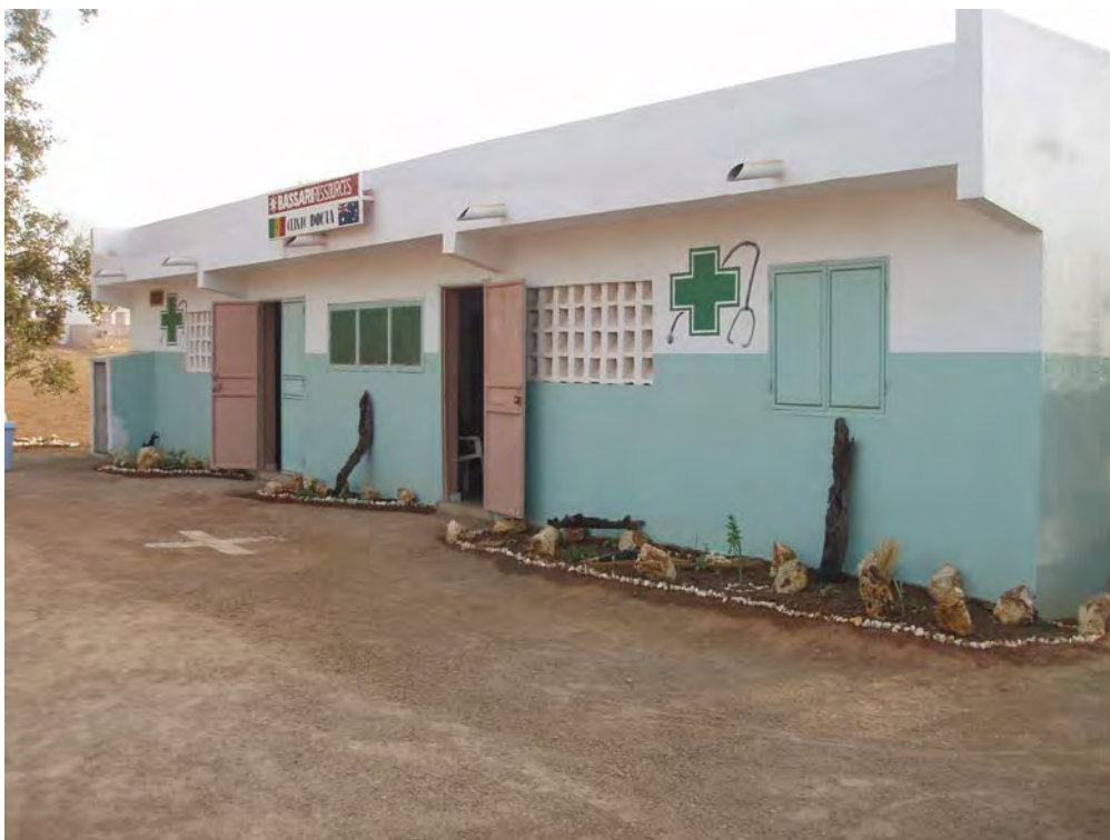
Figure 17 – Douta Medical Centre within Douta Camp compound
