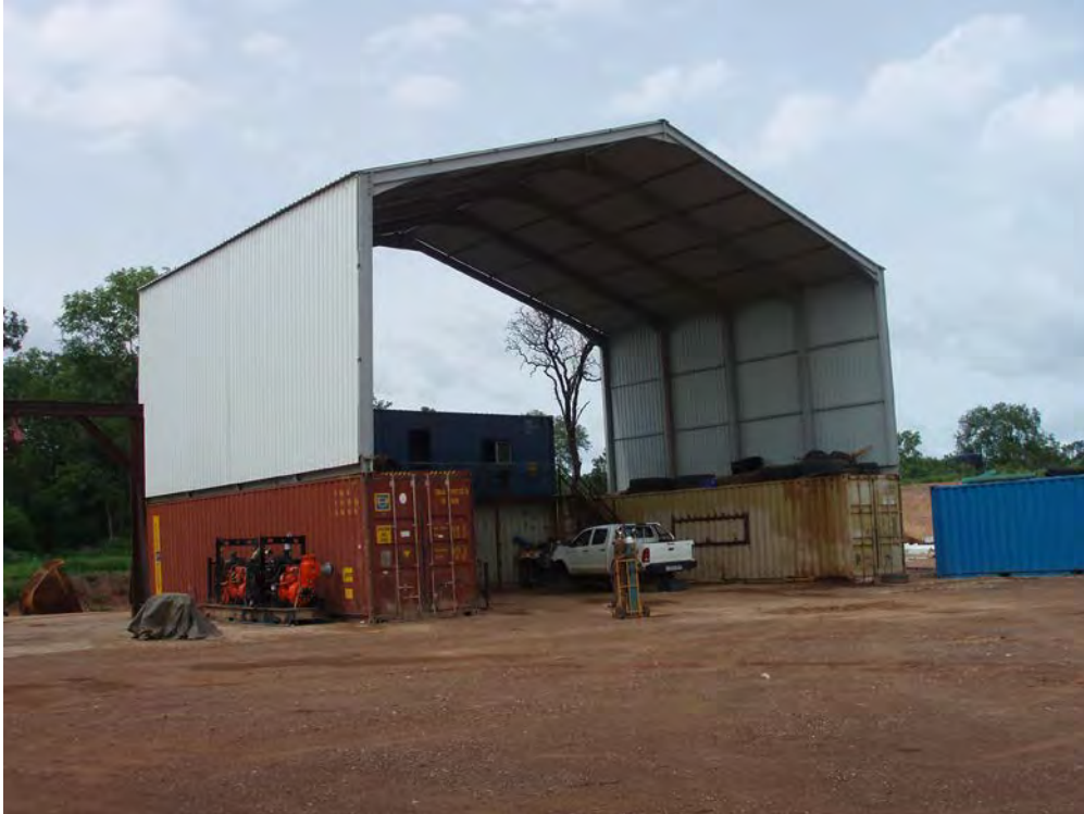
Figure 18 – shows the heavy vehicle maintenance workshop used to service the heavy equipment mobile fleet.
