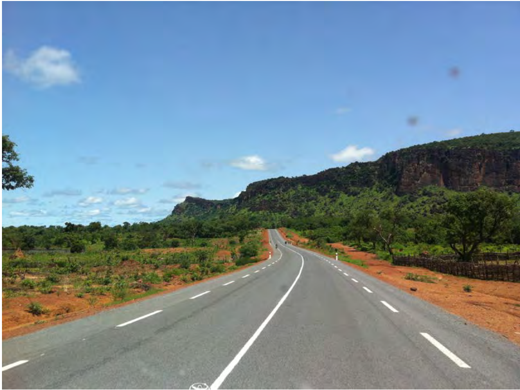
Figure 25 – High Quality Sealed Road from Dakar
