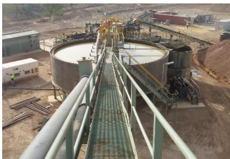
Figure 15 - View of gravity plant from 26 inch cyclone tower
