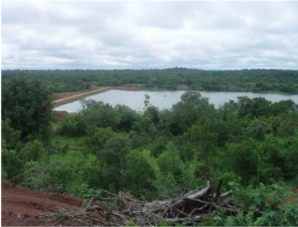
Figure 17 – shows the water storage dam (~500 Megalitres) used for water supply to the processing plant. The dam is currently full.
