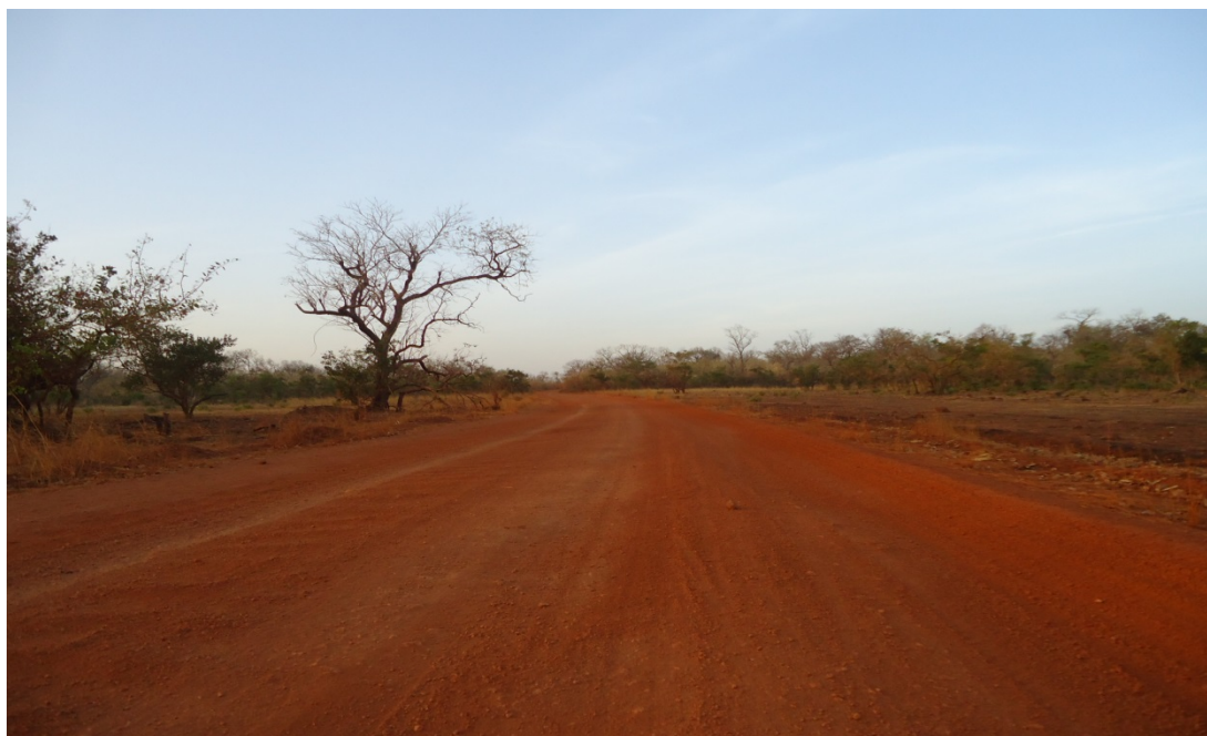
Figure 5 – Existing Road between Makabingui & Processing Facility
