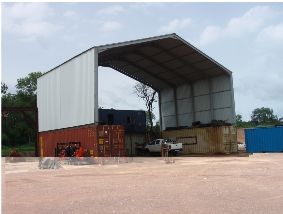
Figure 19 – shows the heavy vehicle maintenance workshop used to service the heavy equipment mobile fleet.
