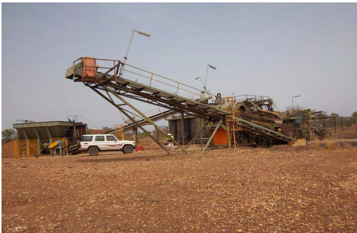
Figure 14 - Gravity Plant Located at Douta – 300ktpa Capacity
