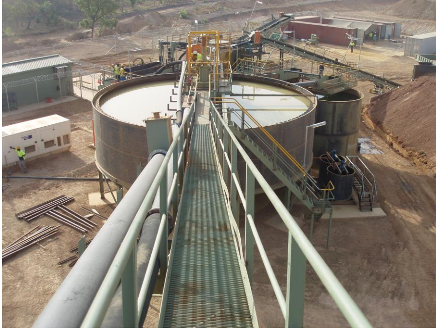
Figure 1 - View of gravity plant from 26 inch cyclone tower
